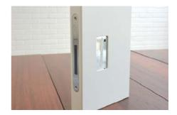
After testing the lock install the <u>finished</u> coverplates.
