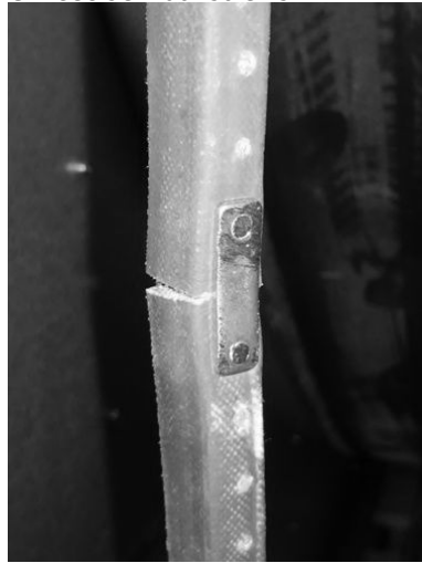
Grinded belt lock screws:
