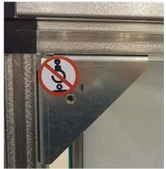
This bracket in Geniox units in the sizes 10 – 18 is not for lifting the unit. This bracket is for permanently holding two sections tight together with 8 mm bolts.
