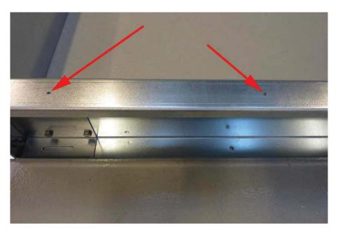
Sections are mounted to base frames with self-drilling screws. In the base frame you will find a sufficient number of 5 mm holes that are prepared for the self drilling screws. In this picture you are standing and you are watching the assembled base frame on the floor or roof.
