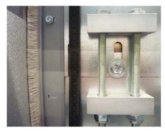
Install sensor for registration of rotation. The sensor must be installed to the right seen from the inspection side of the unit. Check that collision between sensor and brackets at the rotor is impossible. Adjust position of sensor if necessary.
