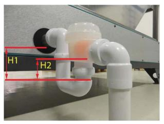
To avoid freeze ups and frost bursts of water trap and pipes, sufficient insulation is recommended and installation of heating between the insulation and water trap/pipes could even be necessary (insulation, heating and controller for the heating are not delivered by Systemair).
