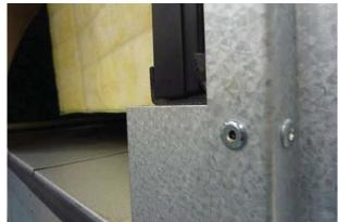
Check that rubber profiles on the back panel as well as rubber profiles on the inspection door are without wear and damage — still sufficient for avoiding any air leakage.
