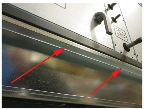
Use self-drilling screws  $-4.8 \times 18 \text{ mm}$  — to be screwed upward through the holes into the bottom profile of the air handling unit **Note!** A screw must be placed in every hole to achieve the necessary strength. In this picture you are lying on the floor or roof looking upward under the base frame. The screws will not be visible, when you are standing beside the unit looking at the unit
