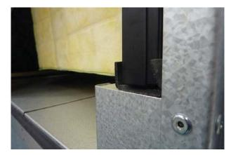
The end of the last filter is fully even with the end of the U-profile. The rubber profile on the inspection door will close the gap between inspection door and filter. Job is
