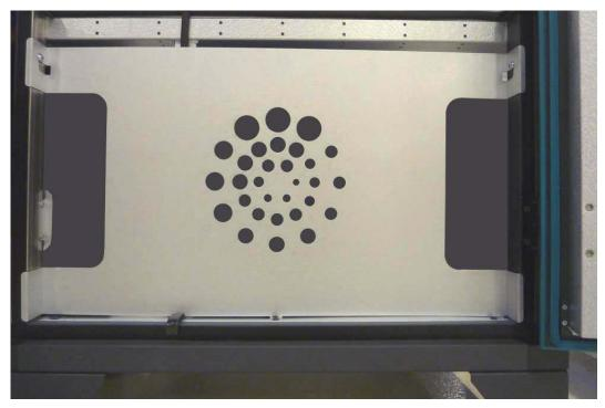
Use an Allan key — size 6 or size 8 — for refitting the safety guard from Systemair. Replace the vibration damping rubber list if it is damaged.
