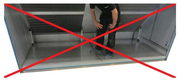
Drip tray with slope is not supported for the weight of a person. Do not walk or stay in the drip tray.
