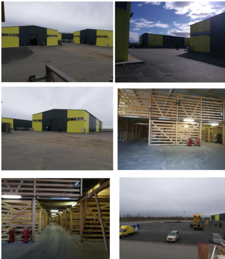
Figure 3. View of the zone and buildings.
