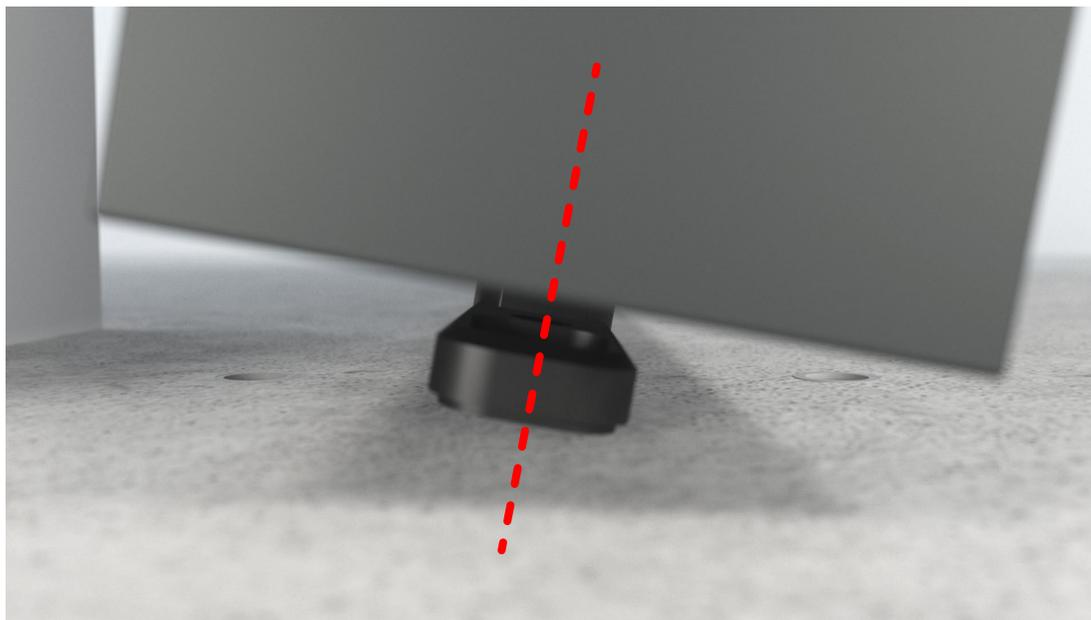
Place the door leaf in the doorway, and position the bottom pivot in between the 2 mounting holes at the axis position.
