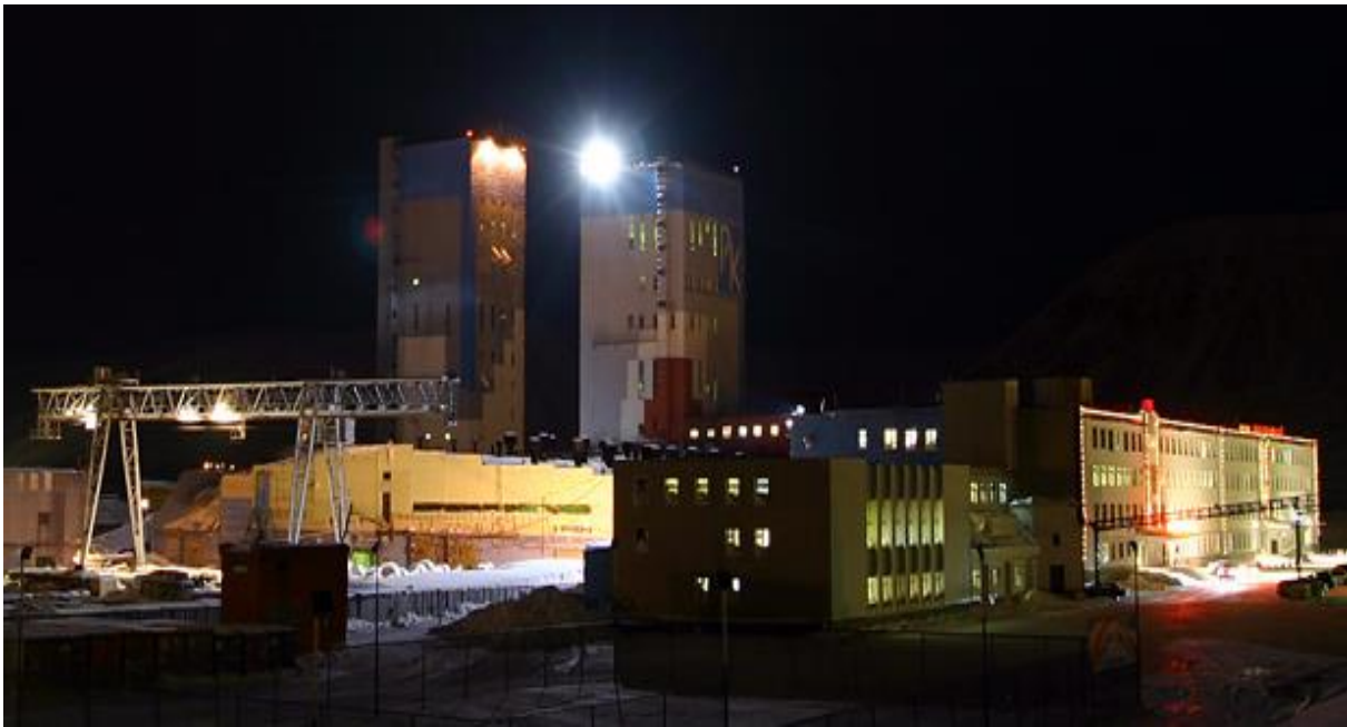
Photo 2. Administrative-household complex of "Komsomolsky" mine
