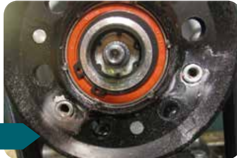
Leaking oil seal
