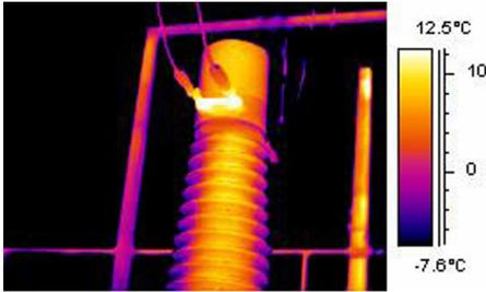
**Figure 25.12** An infrared image of a circuit breaker
