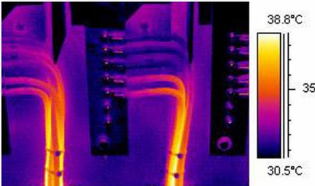
**Figure 25.15** An infrared image of bundled cables
