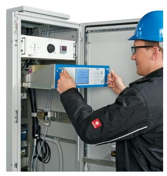
Analyzer and  $\mathrm{NO}_{\mathrm{x}}$  converter are mounted on slide-out racks for easy removal or service.
