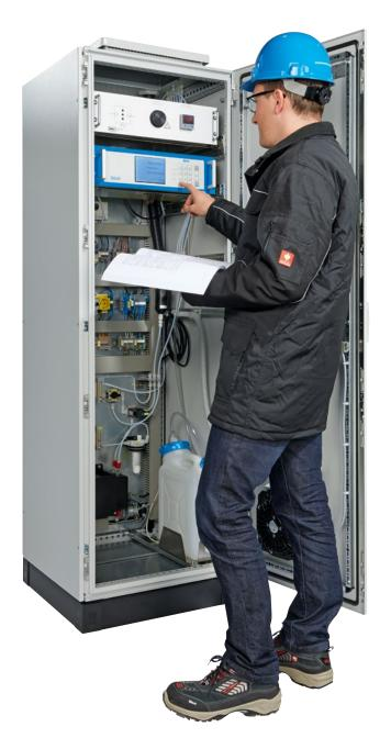
PowerCEMS50 is the newest system in SICK's customized analyzer solution portfolio. The PowerCEMS50 is streamlined to exactly match the requirements of continuous emission monitoring. PowerCEMS50 is designed to continuously and reliably measure emissions from power generating facilities and that's exactly what it's been trimmed down to do.
