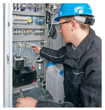
In the PowerCEMS50 the gas wetted components are integrated together in the lower section of the cabinet. This insures that any condensate cannot drip onto electrical components preventing a dangerous and costly situation.
